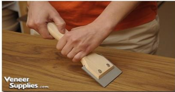
Figure 1: Scraping the veneer is critical to success.
